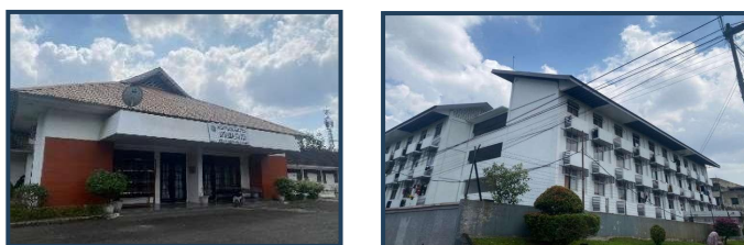
Figure 1 (a) old dormitory building; (b) new dormitory building.
