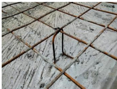
Gambar 8 Pekerjaan Besi Wiremesh
