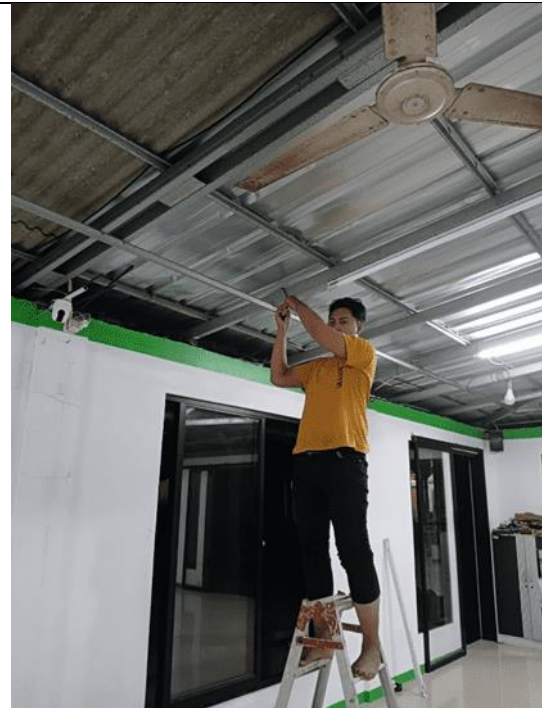
gambar1 21 Proses Pemasangan lampu TL led di area sholat Wanita
