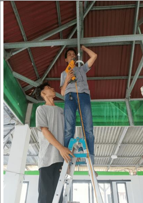
gambar1 16 Proses pemasangan lampu in-lite Outbow
