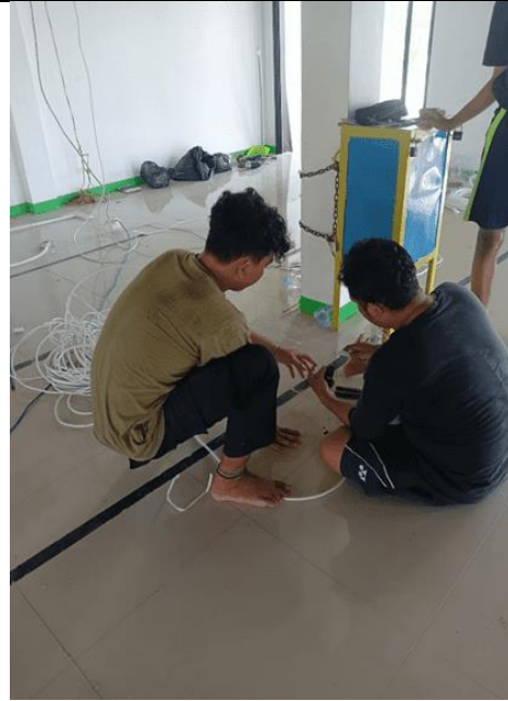
gambar1 12 Proses bending pipa instalasi
