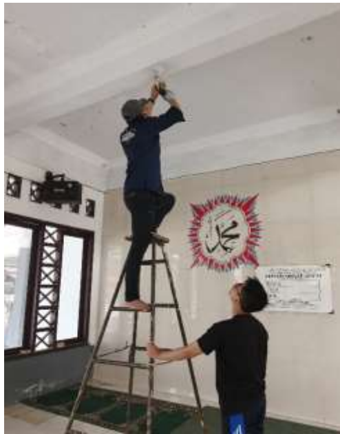
Gambar 6. Pergantian Fitting, Pipa, dan Lampu
