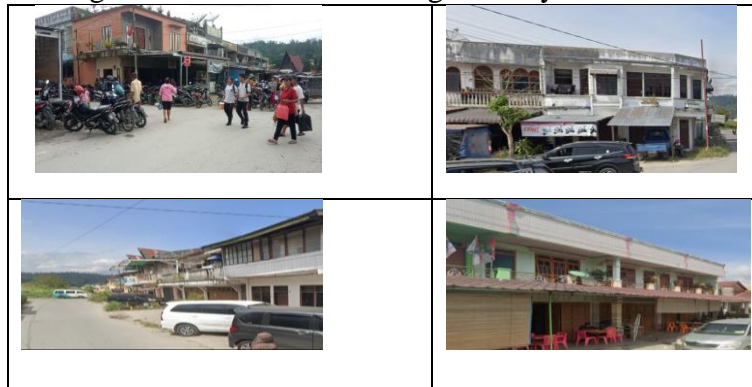
Figure 3 Two-Story Building in the Tarutung Market Area
